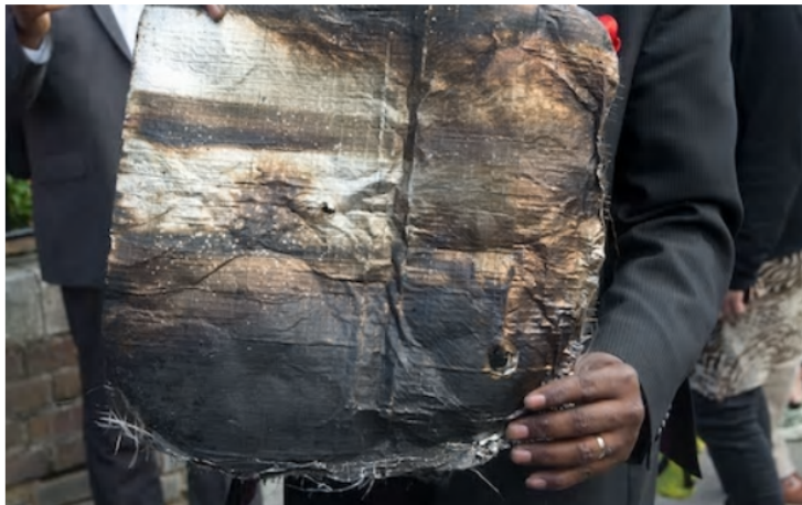
A local residents holds a section of the burnt cladding which fell from Grenfell Tower during the blaze CREDIT: MARK THOMAS/REX/SHUTTERSTOCK
