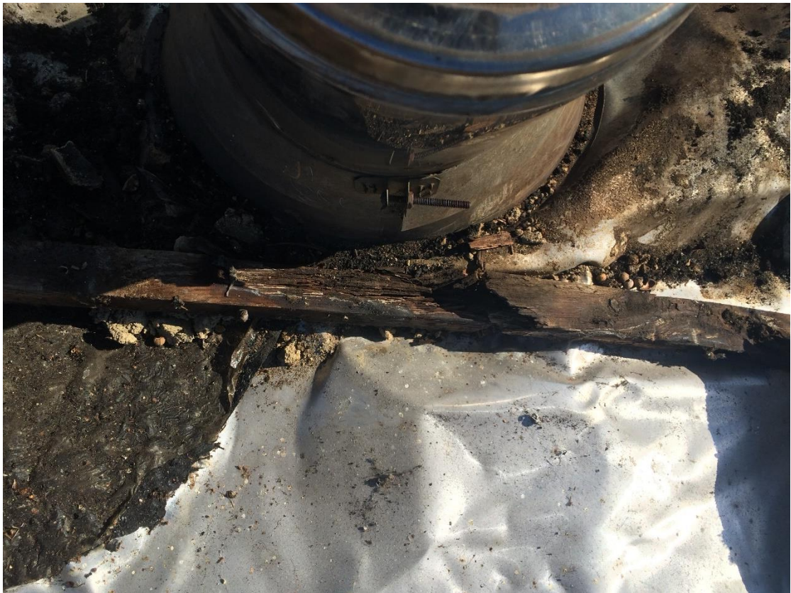
FIRE DAMAGE EVIDENCE
