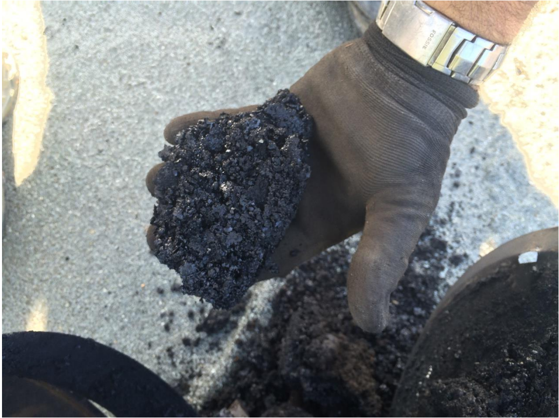
BITUMINIOUS MATERIAL REMOVED FROM FLUE
