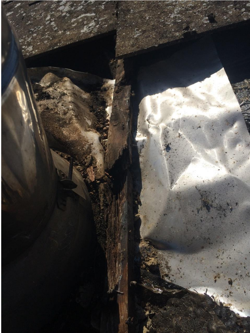
FIRE DAMAGE EVIDENCE AND BITUMINIOUS ROOF FELT
