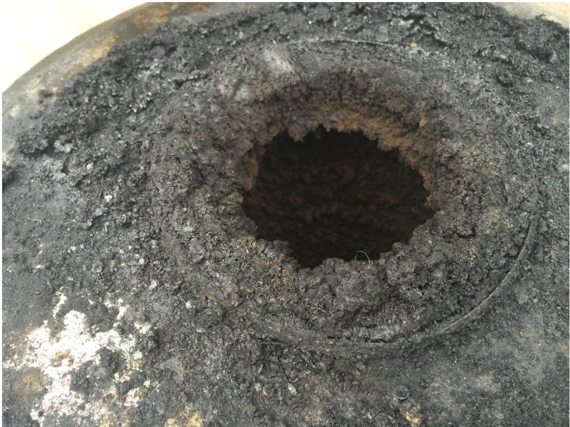
REDUCTION FROM 6 INCH TO LESS THAN 3 INCH
