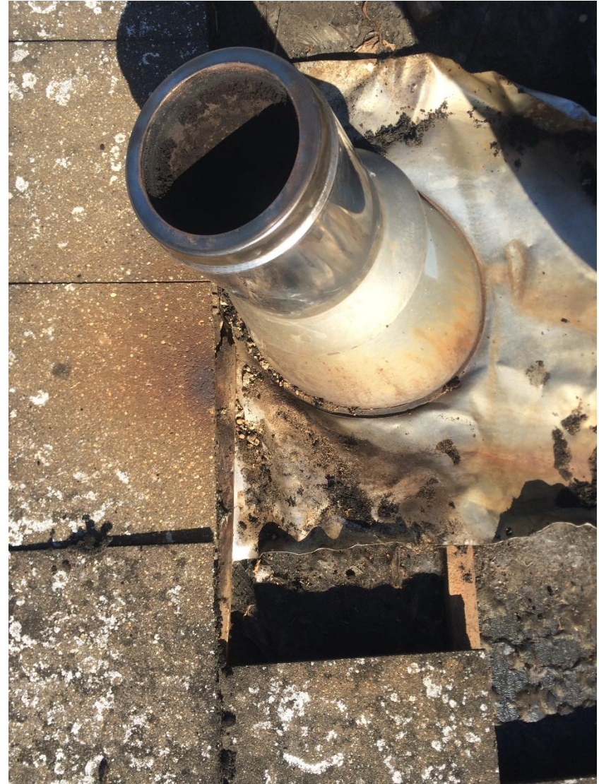
EVIDENCE OF FIRE DAMAGE TO TIMBER BATTEN
