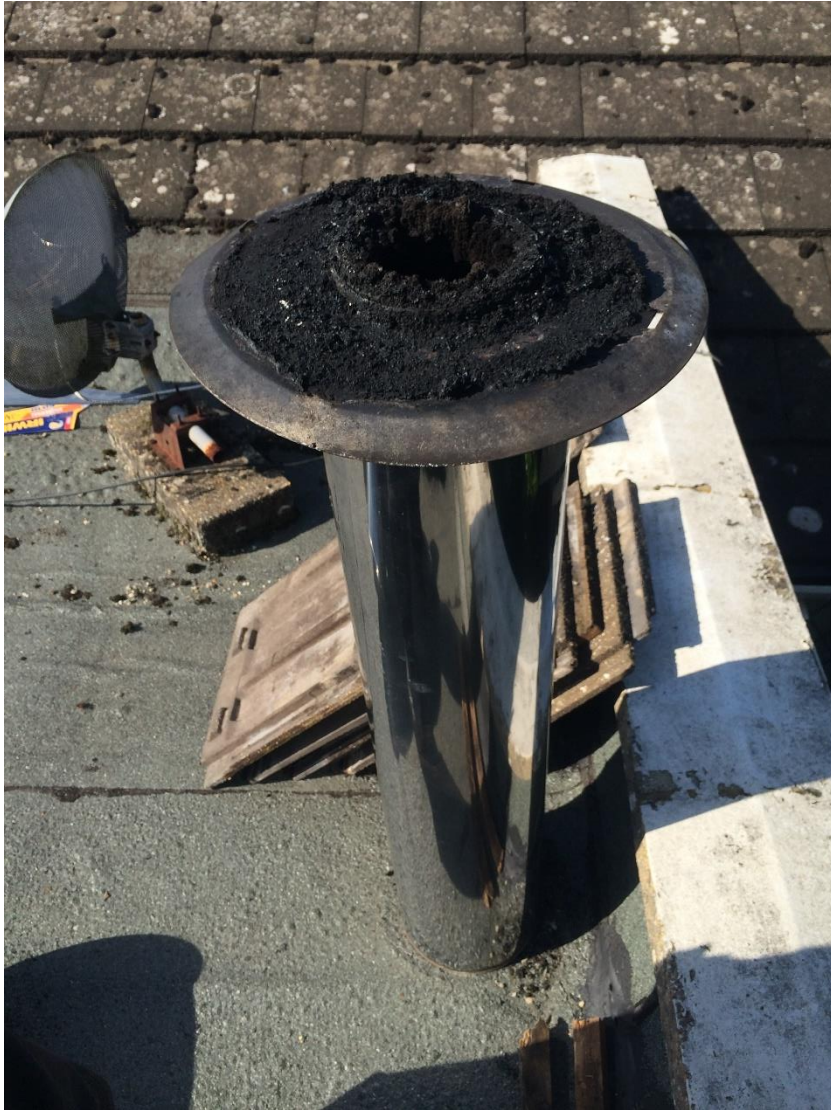
DEFECTIVE CHIMNEY COMPONENT
