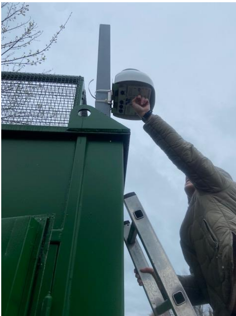
Installing the Kunak AIR Pro PM2.5 sensor
